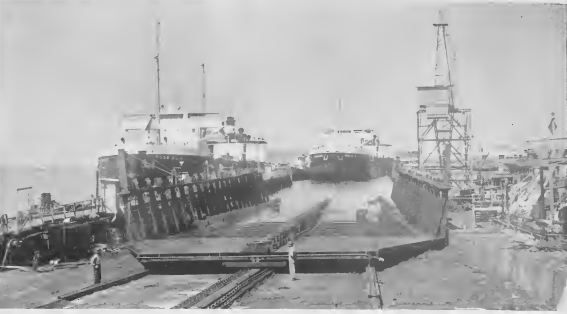
THIS is the Shipyard's Marine Railway made up of the cradle, in front of which the men are standing, and the track upon which it travels. The rollers upon which the cradle moves are shown spanning each track while disappearing down one side of the center track, and disappearing on the other is the chain which moves the cradle. Aligned on the cradle base are the keel and bilge blocks which support the ship.
